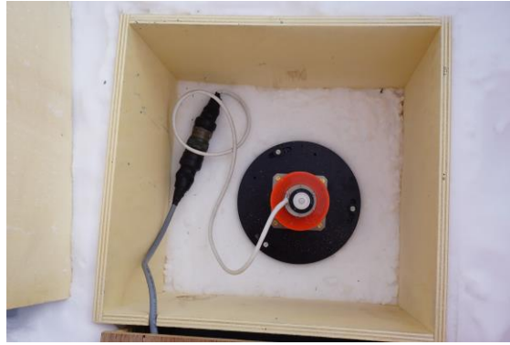
Figure 3. Flux-gate magnetometer sensor installation
