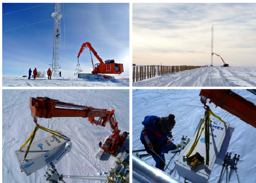
Fig. 6. Installation on the American Tower.
