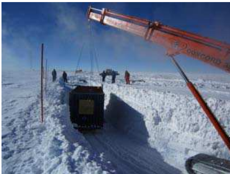
Fig. 2: Burying of the shelter in the snow, the sticks on the left delimit the clean area.
