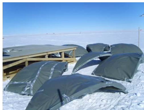
Platform and dome segments after unloading
